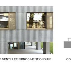
FACADE VENTILEE FIBROCEMENT ONDULE
